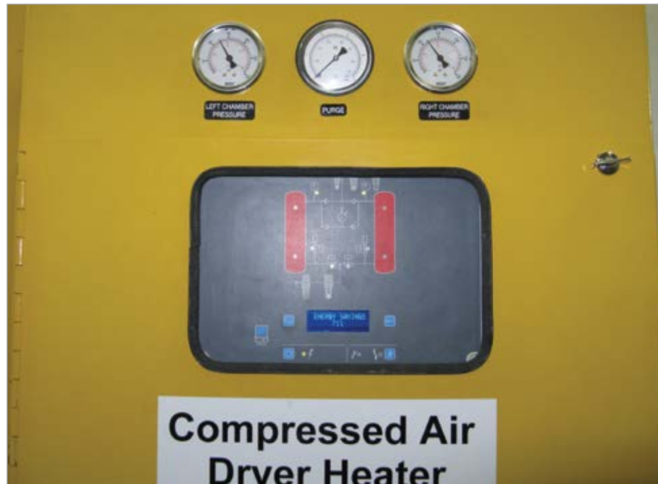
Figure 3: The blower style dryer saves 71 percent due to cool dry conditions and the dew point control.
