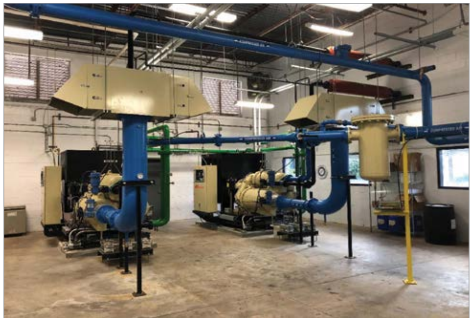
1888 Mills' air compressor room equipped with two Ingersoll Rand C700 Series 600-horsepower Centac centrifugal air compressors.
