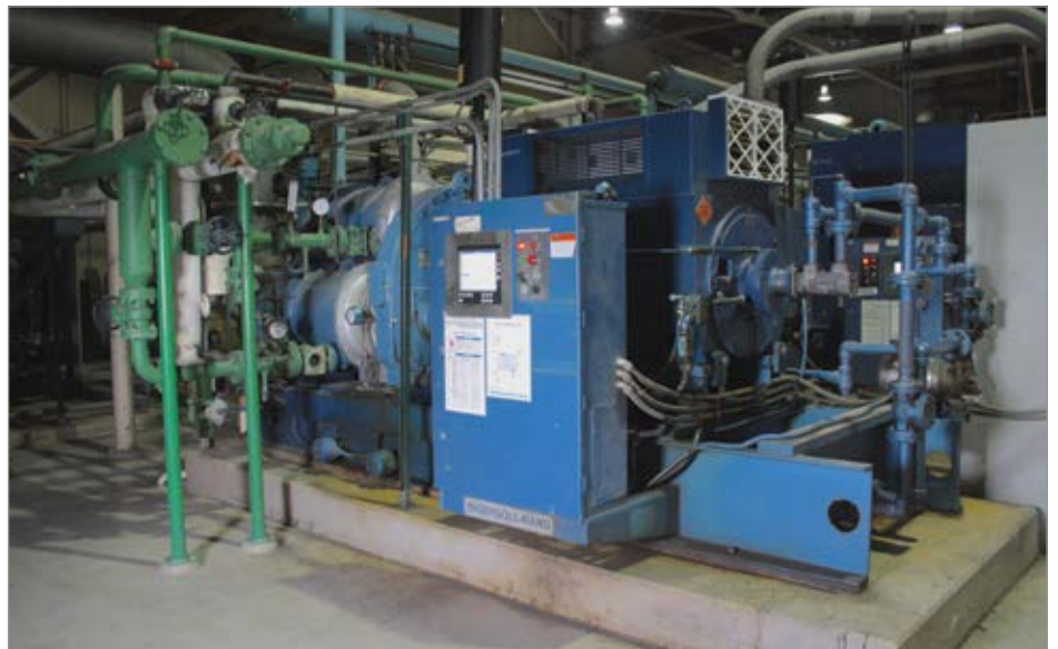
An Ingersoll Rand centrifugal air compressor equipped with a Bay Controls Control System at one of the manufacturer's 10 plants.
