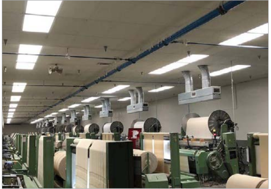
An aluminum manifold provides even air distribution throughout the 1888 Mills facility.
