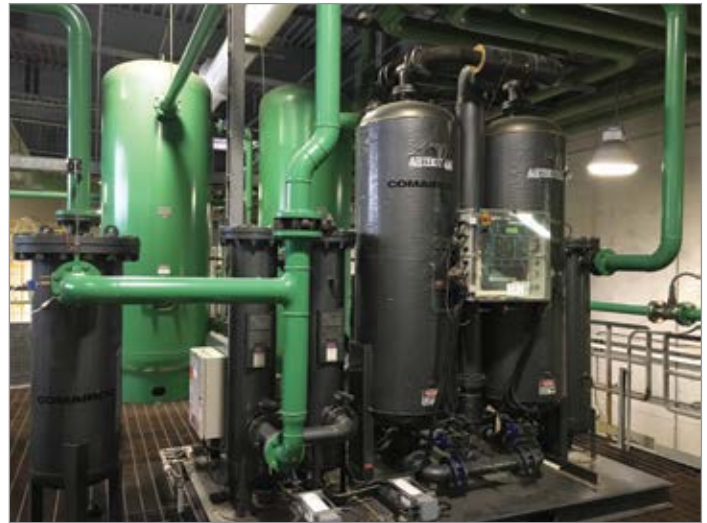
This dryer regenerates infrequently due to lower moisture loading and dewpoint control.
