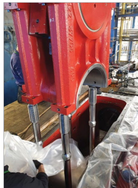
Replacement of bearings and overhaul of connecting rod.
