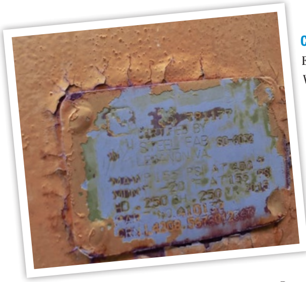
Compressed air storage tank identification plates advise when the last safety inspection took place.
