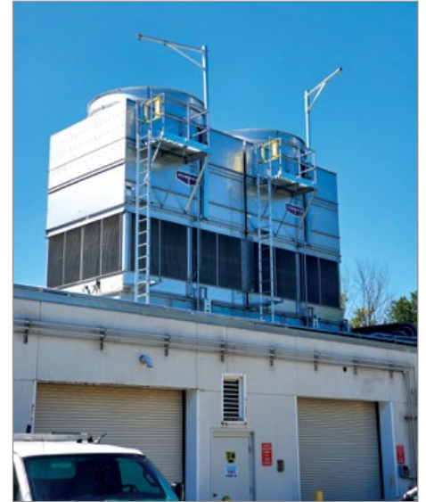
A cooling tower installation Hoffman & Hoffman completed at a local hospital in Greensboro.
