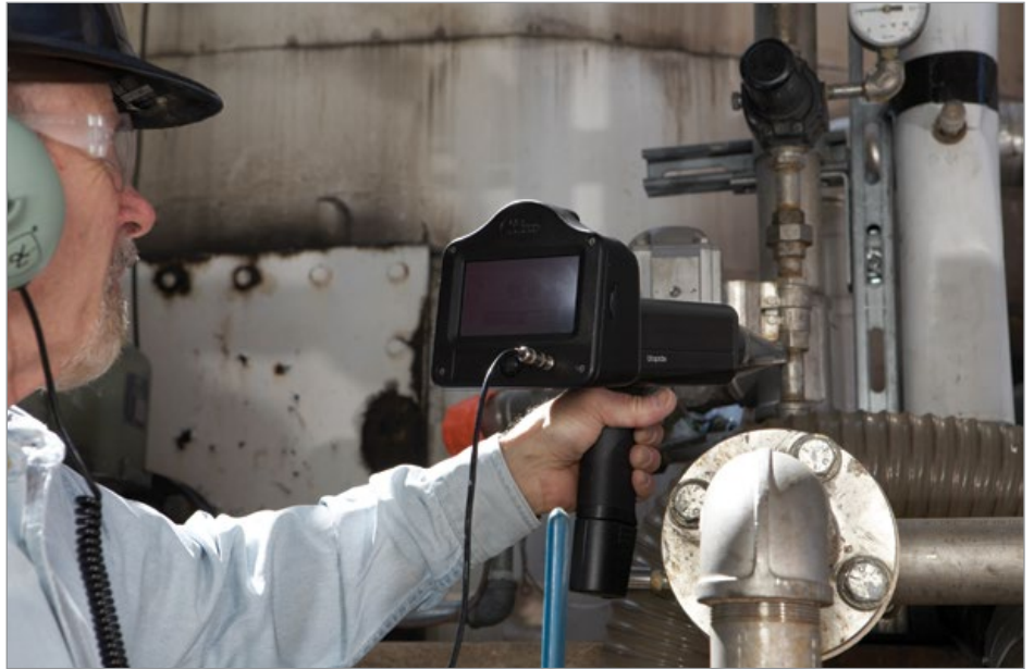
Using an ultrasonic leak detector to identify the source of a compressed air leak.
