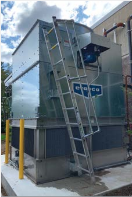
This eco-ATWB hybrid fluid cooler includes a Smart Shield water treatment system, and serves a Massachusetts-based company that does laser powder bed fusion on an industrial scale.
