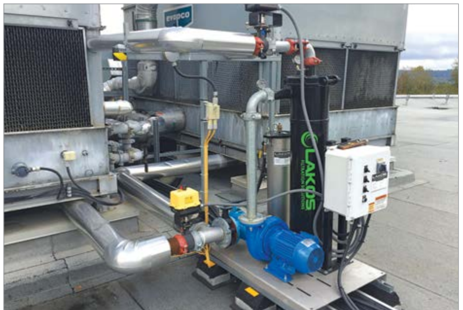
In this installation, a LAKOS basin sweeping system removes debris from a cooling tower basin.
