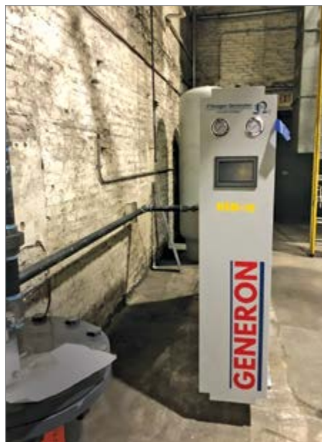
Installing the nitrogen generator
