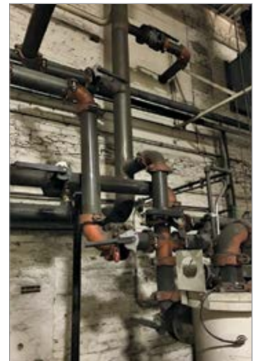
Before the redesign, the compressed air piping configuration was unnecessarily complex.
