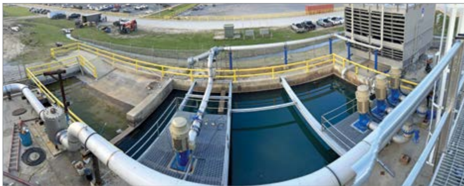
A fisheye view of the pit and its three sections
