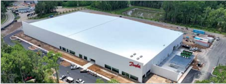
Danfoss Turbocor's expanded production facility, which doubled manufacturing capacity with the ability to expand even further, opened in May 2024.
