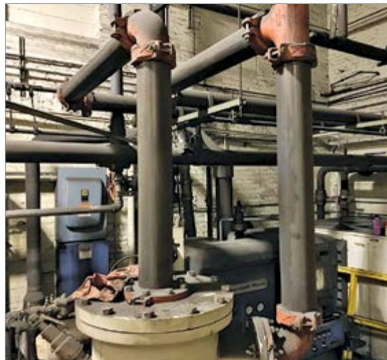
Before the redesign, the compressed air piping configuration was unnecessarily complex.
