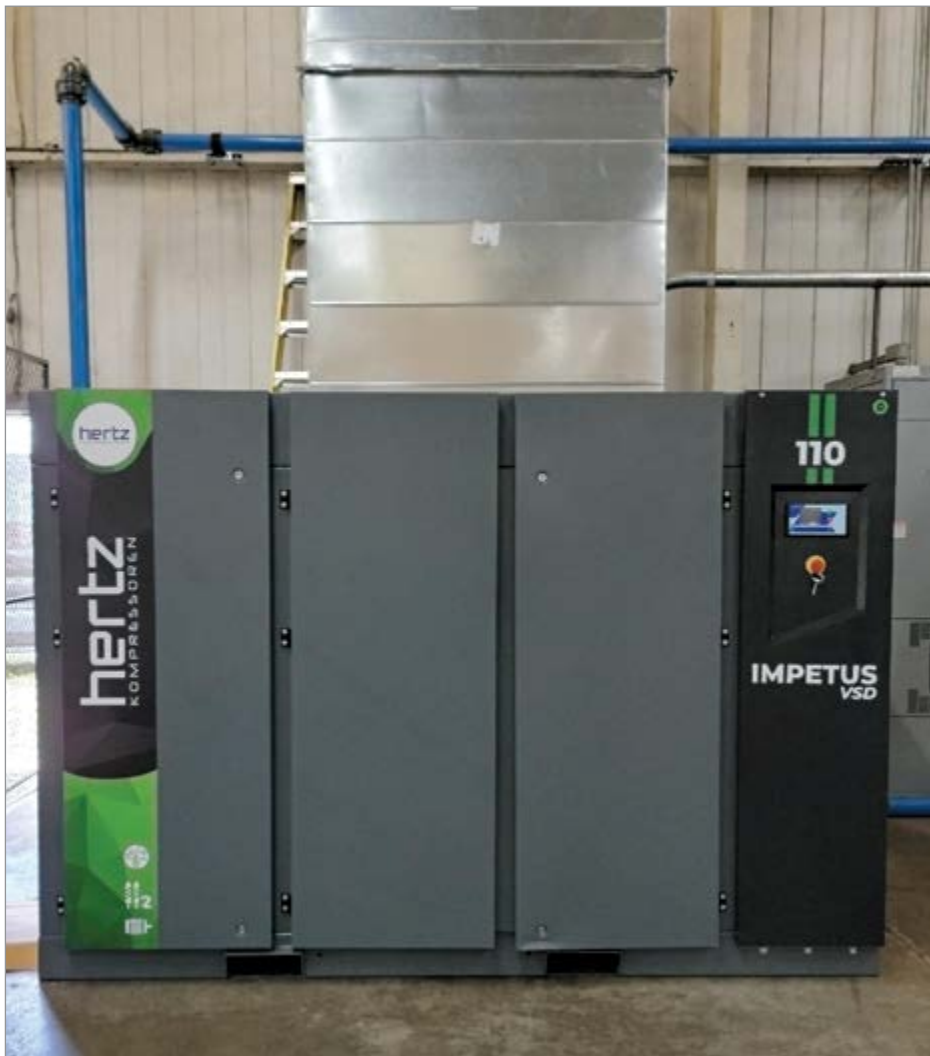
A Connecticut manufacturer of steel, plastic and fiber drums, as well as other packaging products, installed a two-stage 150 hp variable speed rotary screw air compressor to save energy and create a heat recovery system.
