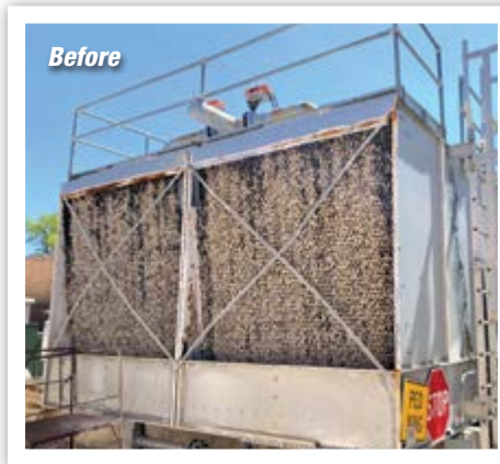
This crossflow cooling tower looks new again following a full fill replacement.
