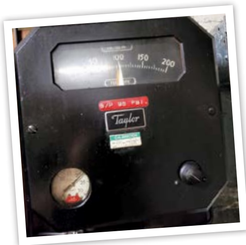
Replacing this pressure controller with a newer and more accurate model should have a quick return on investment.
