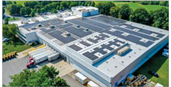
The solar systems at Kaeser Compressors' U.S. headquarters in Fredericksburg, VA, are set to generate over 1.2 million kilowatt-hours of clean energy annually, significantly reducing the facility's carbon footprint.
