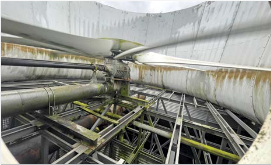
A porthole view of one of the fans atop the main plant's induced draft cooling towers.
