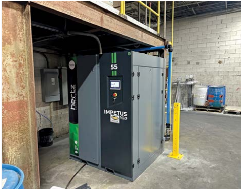
A 75 hp two-stage rotary screw air compressor was installed at an anodizing and impregnating company in Illinois. The customer is realizing 10% more compressed air with a 10% energy savings compared to the 75 hp VSD air compressor it replaced. This air compressor was sold and installed by Compressor Services of Johnsburg, IL.
