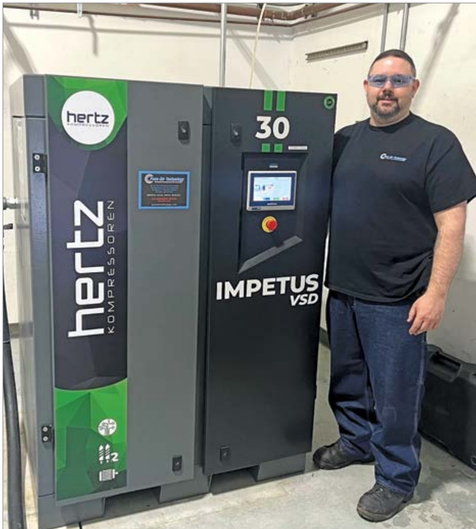
Jared Lambert, owner of Pneu-Air Technology, replaced two air compressors – a 25 hp and a 30 hp – with a 40 hp two-stage air compressor at a Connecticut chemical manufacturing plant. The two-stage air compressor produces more air than the two air compressors it replaced while using 15% less energy.
