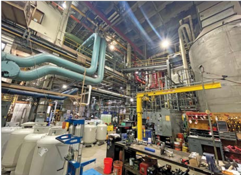
Color-coding the pipes helps the Minneapolis district energy main plant stay organized. The area where employees perform chemistry testing is in the front.
