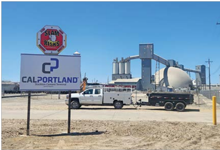
Stockton West Cement terminal in California
