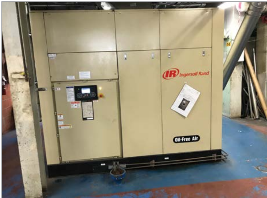
An oil-free rotary screw air compressor at the Molson Coors Toronto Brewery.
