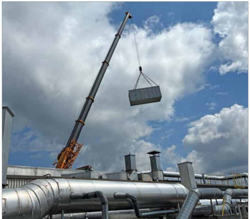
Coordinated rigging and crane work was essential to set and assemble the makeup air unit.
