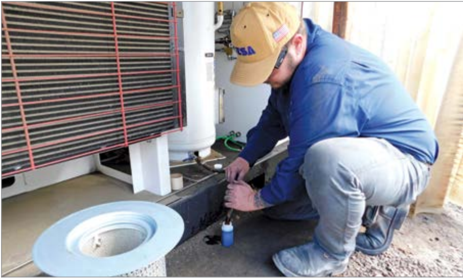
A technician takes an oil sample for lab analysis, a proactive diagnostic measure used to monitor lubricant condition, detect early-stage wear and extend air compressor service life.
