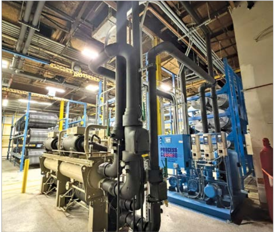
A central heat recovery equipment circulates fluid between the house chilled water system and the recovery system.
