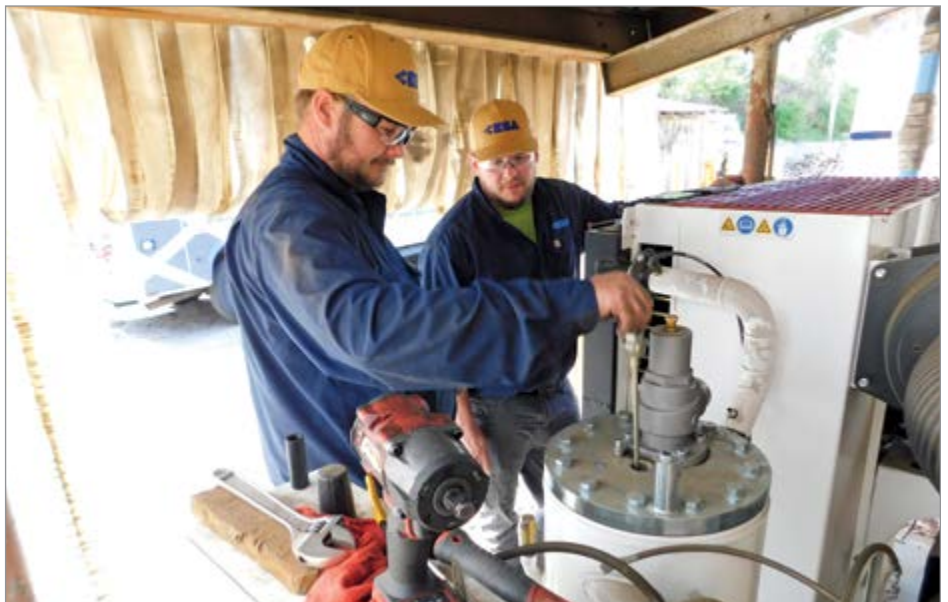
A technician performs an oil separator element changeout on an oil-flooded, rotary screw air compressor as part of a scheduled preventive maintenance service.
