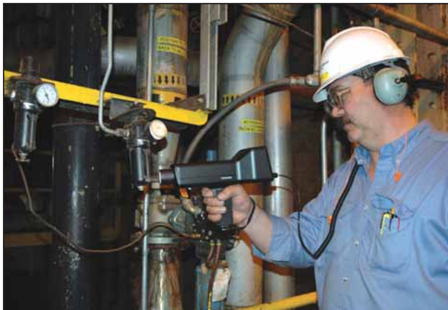
Ultrasonic leak detectors with digital read-outs are effective tools.
