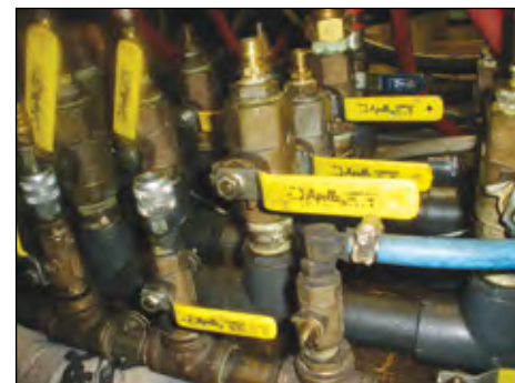
Air leak on hose/fitting connect
