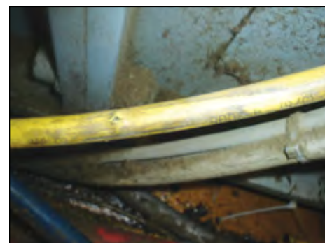
Multiple holes/leaks in tubing
