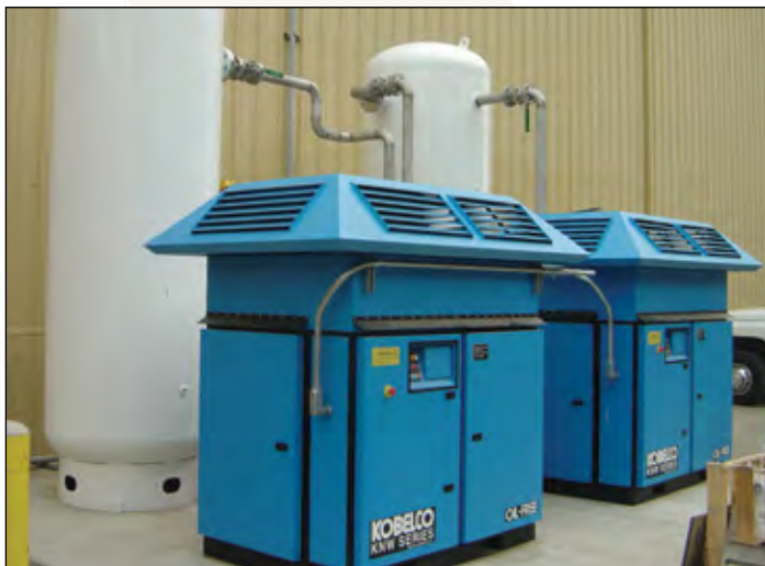
Oil-Free air compressors at a food processing plant.
