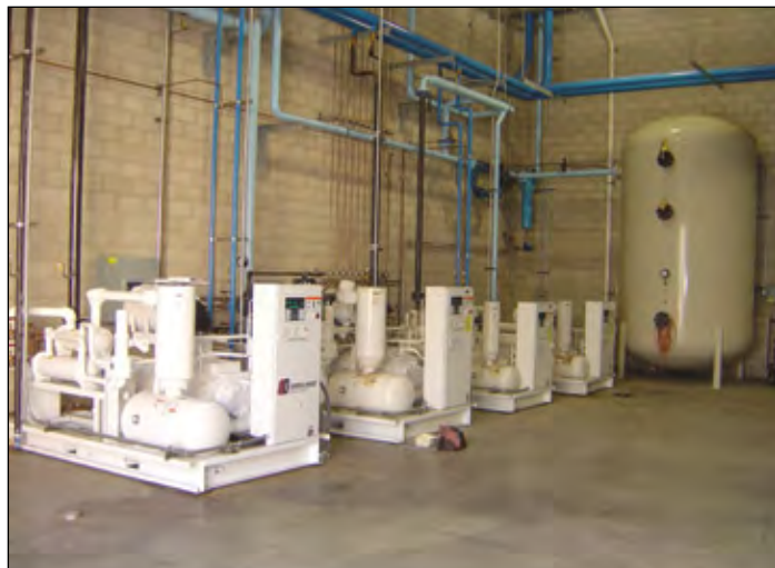
Air compressors with automated sequencers and air storage save energy at a farm in central California.
