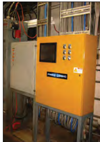
A Pneu-Logic Master Controller Installed at a Lumber Mill
