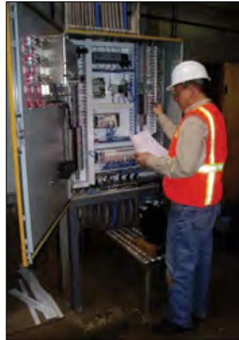
Eric Bessey, Chief Project Engineer for Pneu-Logic, configures a PL4000 Master Controller
