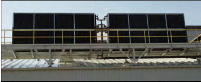
A Large Dry Cooler System
