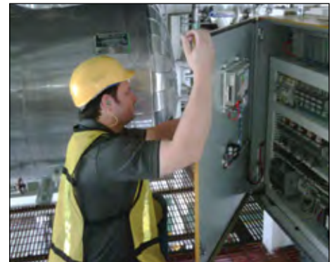
Dusty Smith of Pneu-Logic tunes a PL4000 compressor management system
