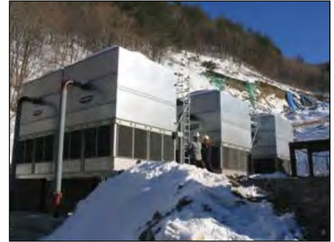
A Closed-loop Evaporative Cooler System
