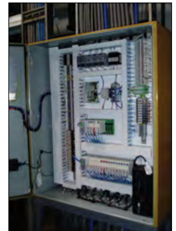
A Pneu-Logic Master Controller Installed at a Lumber Mill
