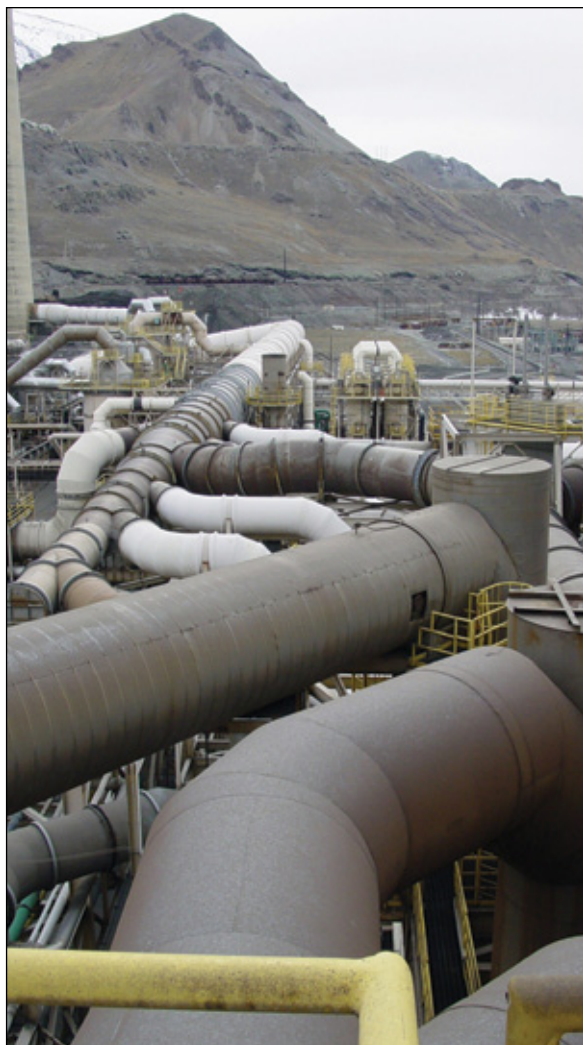
Retrofits to Fume Filtration System at precious metals smelter cuts use of compressed air by nearly 70%.
