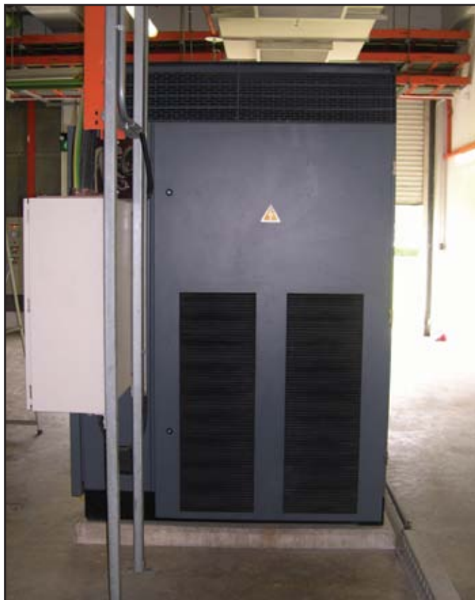
The air compressors were experiencing air intake temperatures above 100 °F. Installing exhaust ventilation duct work on the air compressor helped lower ambient temperatures in the compressor room.
