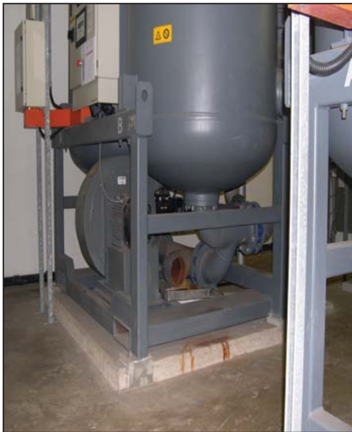
The desiccant air dryer was exhausting 230 °F hot, humid air into the compressor room during the 4-hour regeneration cycle.
