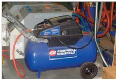
Small dedicated compressors are used for chemical tanks
