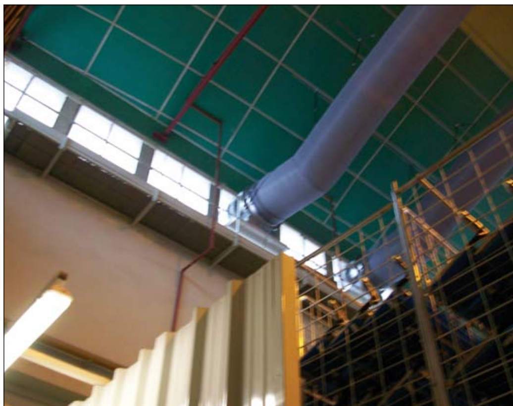
Installing fresh air ducting improves positive pressure in plant and off-sets heating requirements
