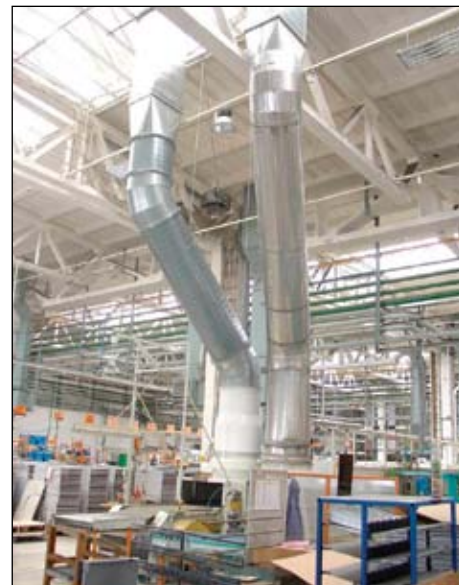
Furnace make-up air is supplied directly from outside to improve pressure balance and reduce heating requirements
