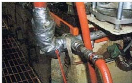
Figure 1A. Some leaks are easy to spot – Look for the duct tape
