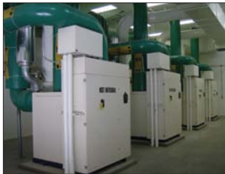
Gearless Turbo Blowers installed at the Fond du Lac plant. (Courtesy ABS USA)
