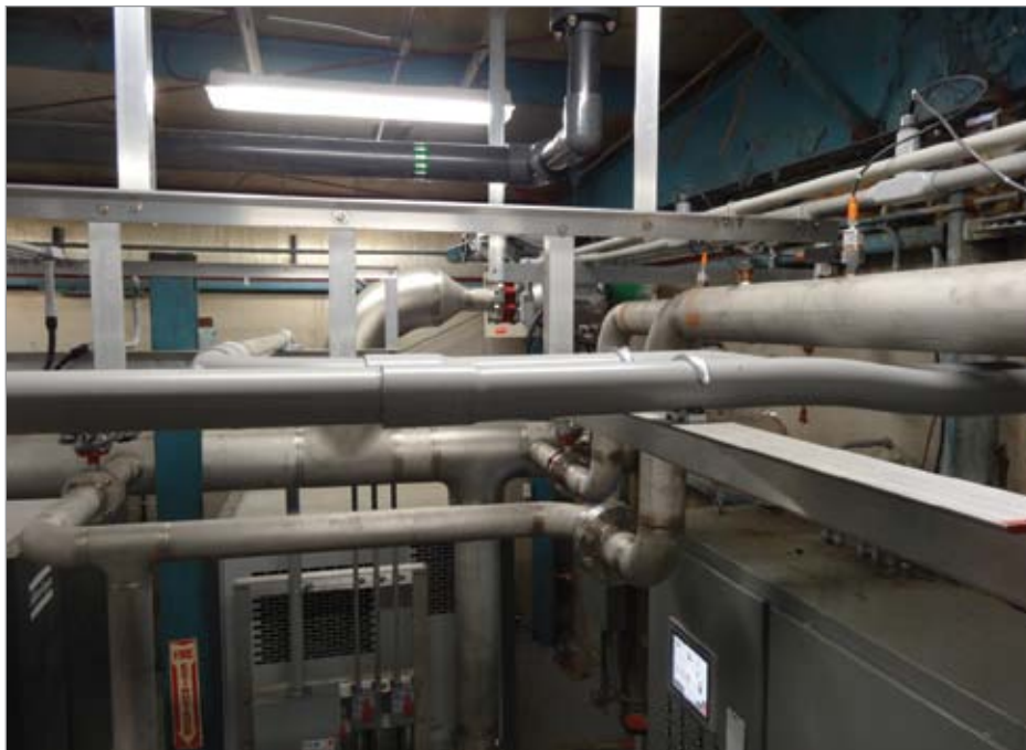
This custom piping solution delivers 7-8 psig air to four biological treatment processes.
