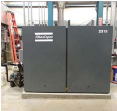
The Atlas Copco ZS 18 is a 25 horsepower oil-free positive displacement rotary screw blower featuring a state of the art oil-free screw element, integrated gearbox and TEFC IP55 motor.
