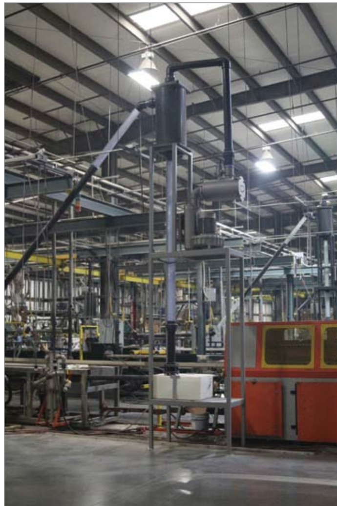
The water separation system for the dry pumps at the tank line.
