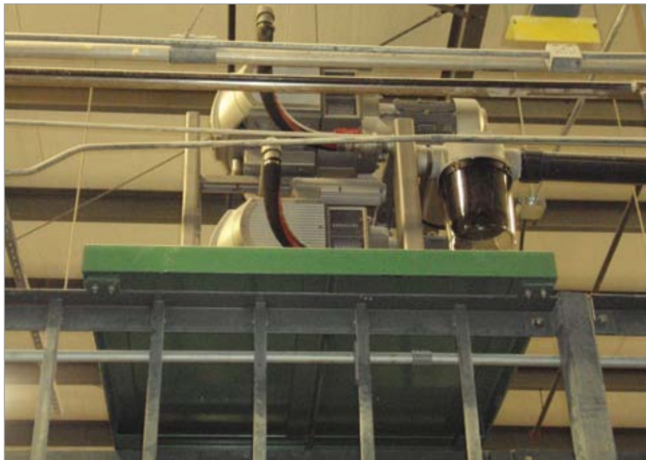
The tandem fixed-speed and VSD Becker dry rotary vane pump system.
