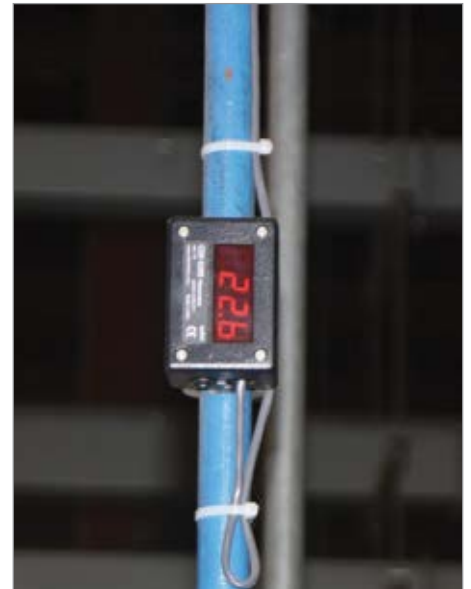
CDI 5200 flow meter serving an individual piece of equipment in a ceramics manufacturing plant
