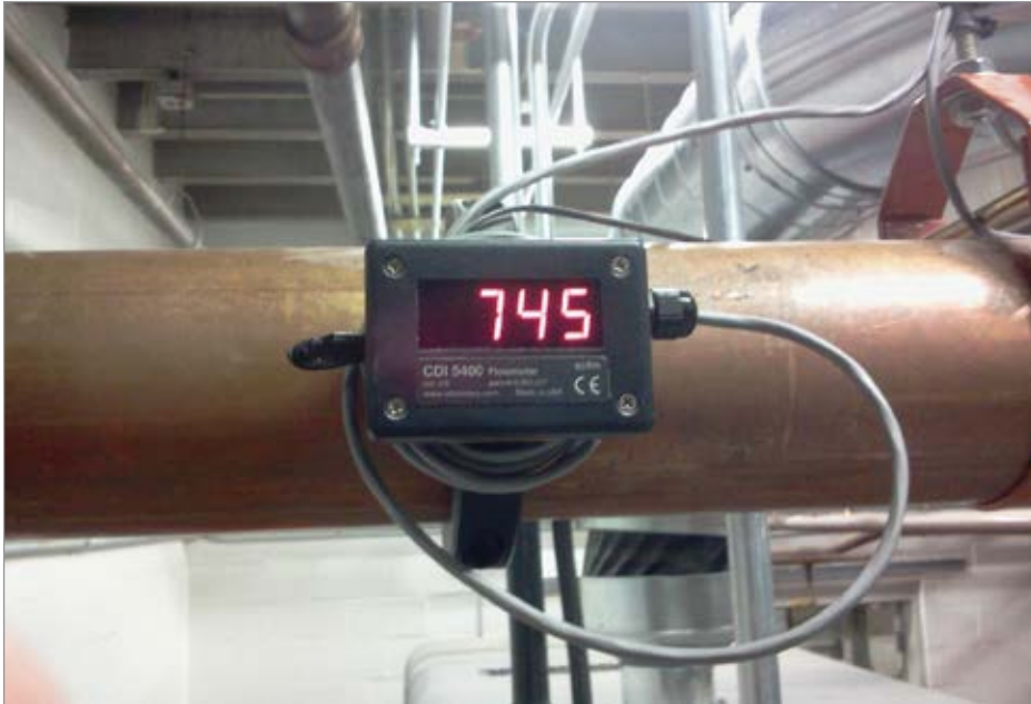
CDI 5400 flow meter installed on a major air distribution line in a lamp manufacturing facility
