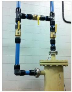
Figure 7: Mist eliminator filter and associated piping
