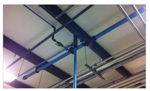
Figure 3: Aluminum piping system — The aluminum pipes are blue in color and slip fit connectors are black.
