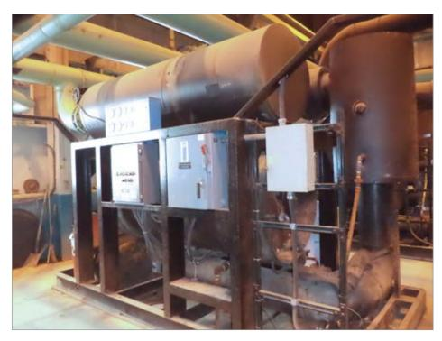
Figure 3: Hybrid-style dryers are used onsite to condition the air for the smelter. This is the 10,000 cfm rated refrigerated part of the combined refrigerated/heated/blower desiccant unit.
