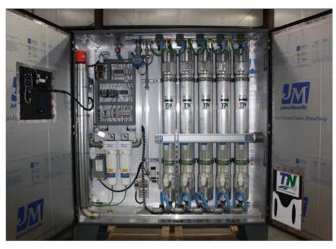
Figure 4: Custom-engineered nitrogen generator that stages from one to five modules
