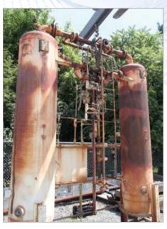
Figure 1: The refinery's original ORIAD© Series internally heated reactivated dryer after years of disuse
