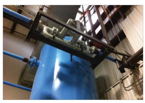
Figure 5: Pressure/flow controller regulating plant pressure to 85 psig (bottom view with tank shown)
