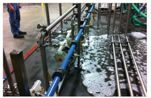
Figure 4: Diaphragm pump header regulated to 55 psig
