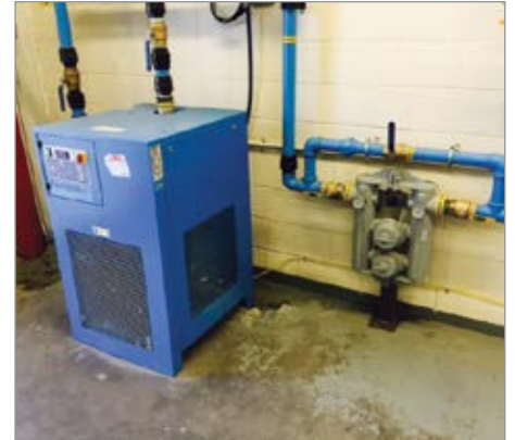
Figure 3: Refrigerated dryer connected to aluminum piping
