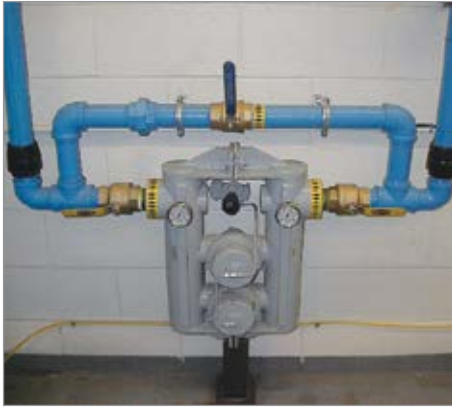
Figure 4: Compressed air flow regulator
