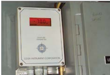
Figure 2: Dew point on this dryer was always a rock solid -70°C.
