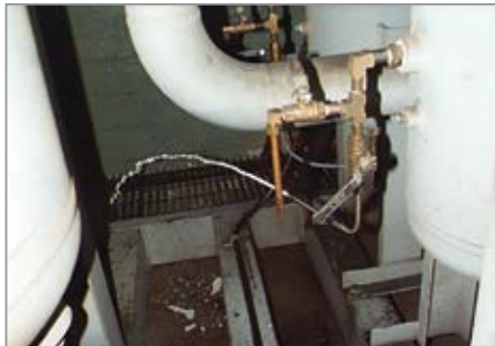
Figure 3: A check on the dryer after filter showed the -70°C reading was in error.
