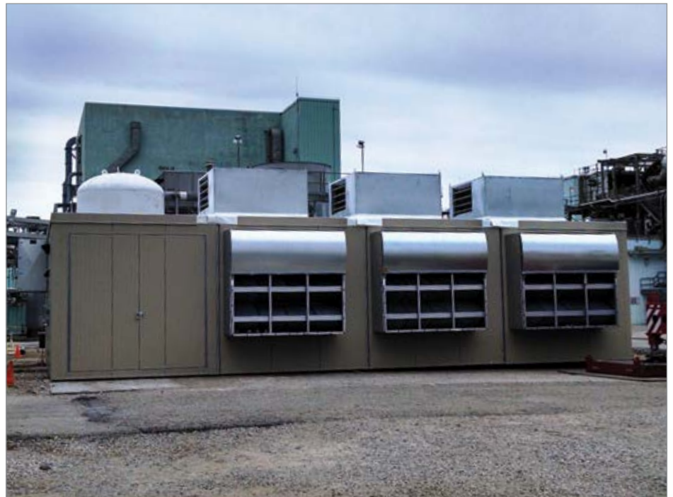
The DirectAIR® installation, including three oil-free rotary screw air compressors
