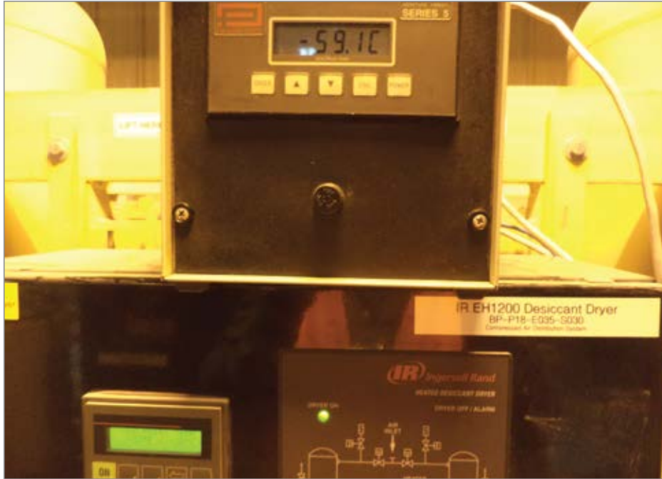
Figure 1: A check against a portable meter (top center) shows a 22°F difference from the onboard probe.
