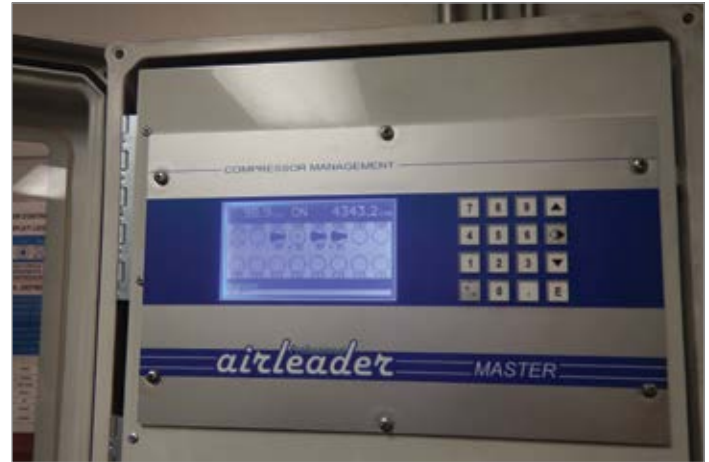
Figure 5: This controller runs the air compressors with best efficiency at full load and varies the flow of the compressors with variable capacity control.
