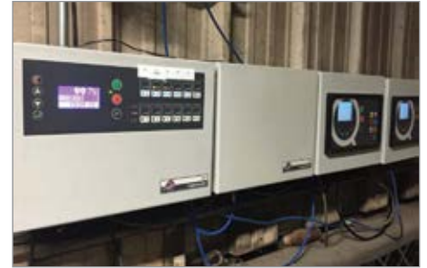
After the commissioning of the Metacentre XC, the pressure band was maintained within 10 psi (vs. 25 psi before).
