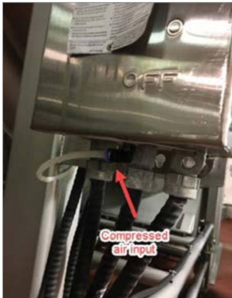
Figure 4: Numerous compressed air connections have been added to electrical panels.
