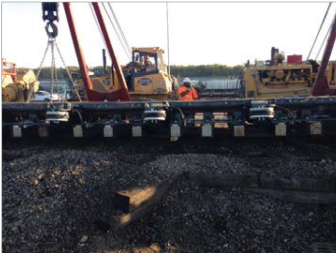
The new compressed air piping system being cutover to the retarders at Alton & Southern Railway.
