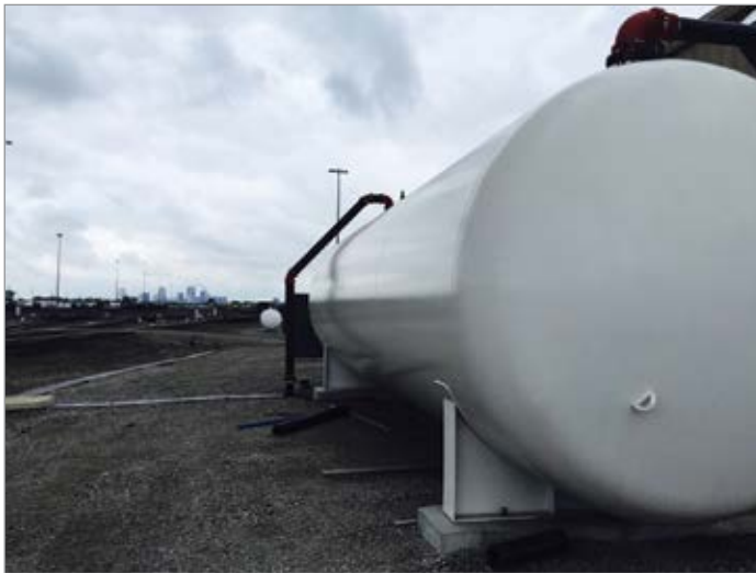
One 5,000-gallon compressed air tank located at the top of the hump yard where demand from the retarders is greatest.
