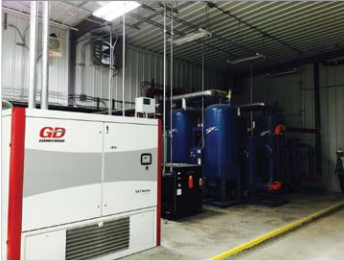
The new heated purge desiccant dryers located inside the air compressor building.
