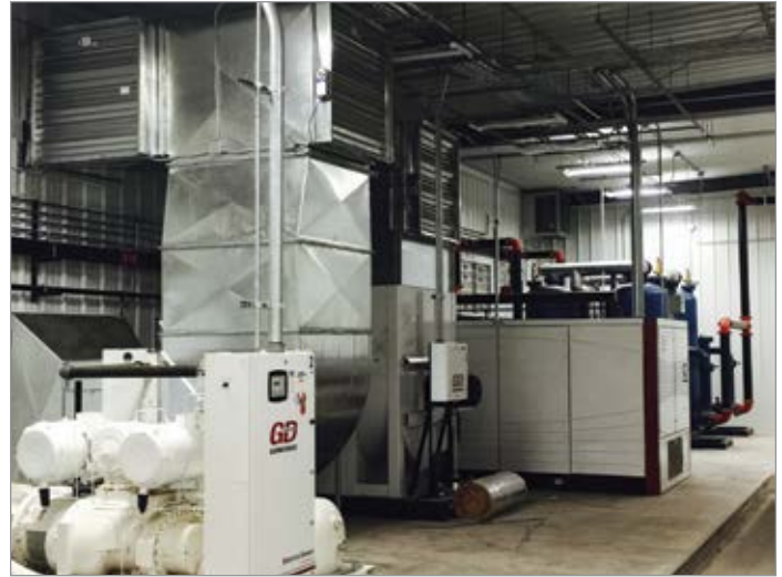
The VSD air compressor handles the intermittent demand, from the retarders, very efficiently.
