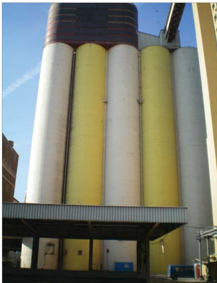
BOGE BLUEprotect is based on the principle that pests that threaten grain stored in silos cannot survive without oxygen.
