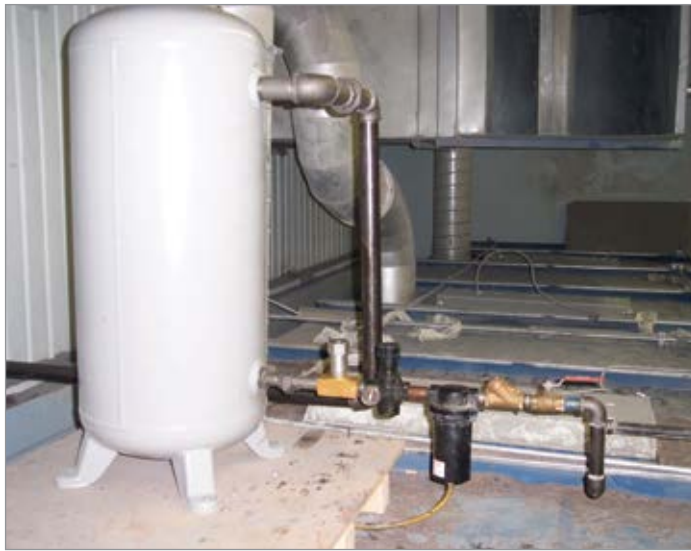
Figure 5: This flow-restricted receiver was installed at the garment plant to solve the problem of transient airflows that were starting a second air compressor.
