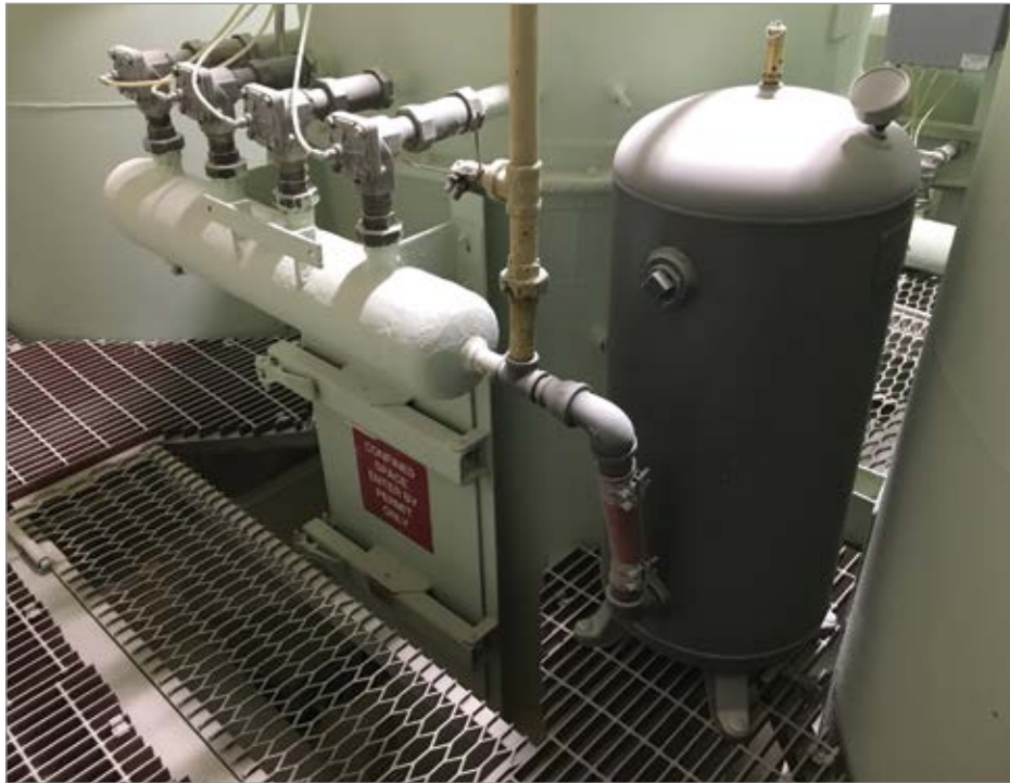
Figure 2: A 60-gallon receiver was added to each problematic dust collector to provide more available compressed air volume per cleaning pulse. The extra storage provided a noticeable increase in pulse strength, popping the bags better for cleaning.
