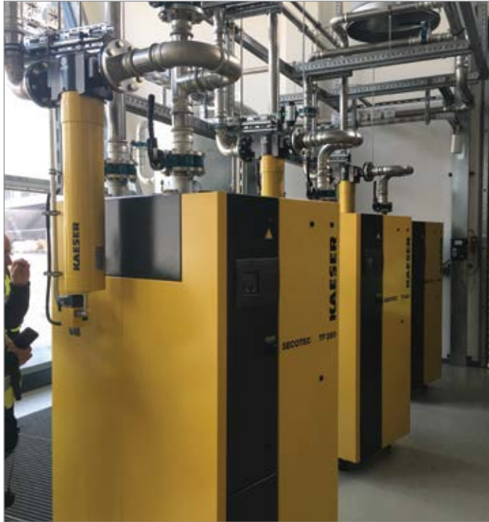
Kaeser compressed air refrigerated dryer technology, featuring R-513a refrigerants with a low Global Warming Potential (GWP) of 631, installed at the Kaeser world headquarters in Coburg, Germany.
