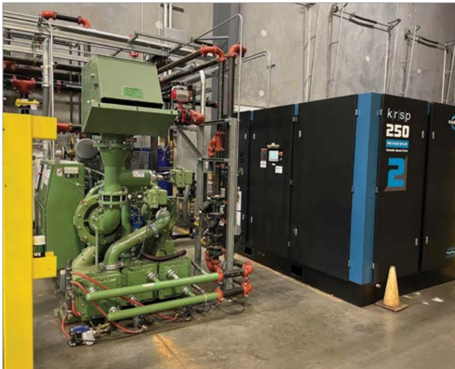
An air compressor room with centrifugal and two-stage rotary screw air compressors.
