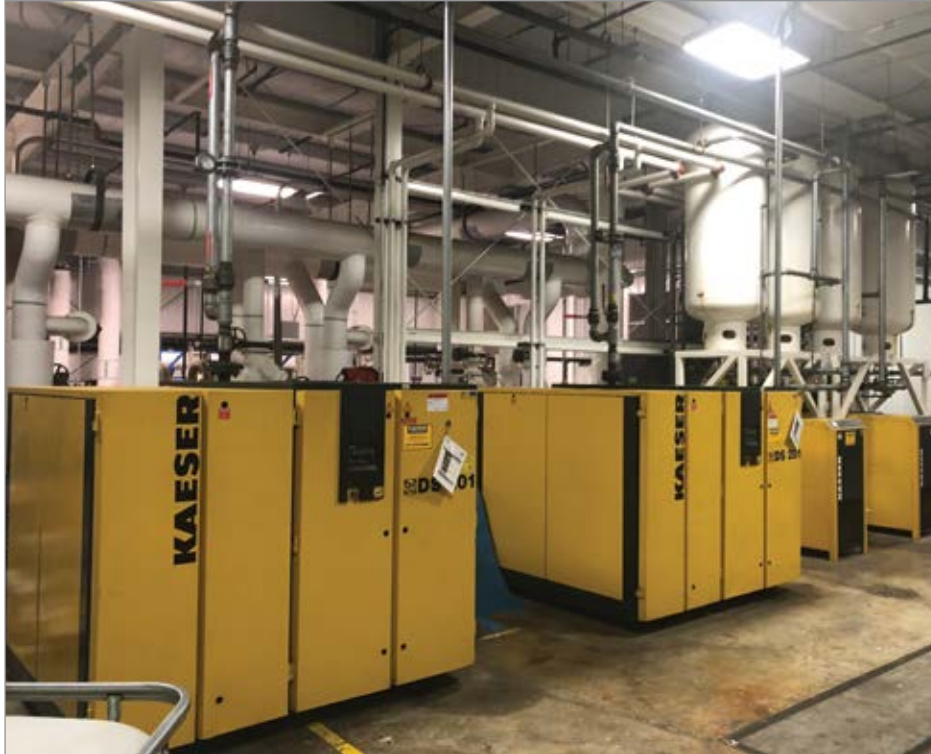
An air compressor room with single-stage rotary screw air compressors and refrigerated compressed air dryers.
