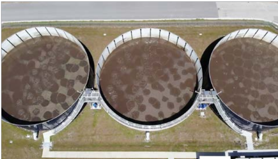
Figure 3: Short-duration bursts of compressed air mix an area of the tank 2-3 times per minute.
