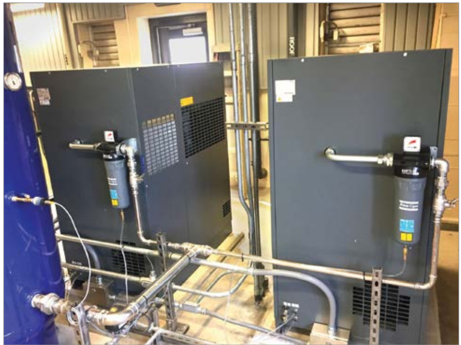
Figure 6: Low-maintenance compressor system matches mixing air demand with duty and standby configuration.
