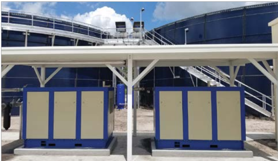
Figure 4: Compressors under a canopy meet the process mixing air demands of the BioMix system for all three equalization tanks.
