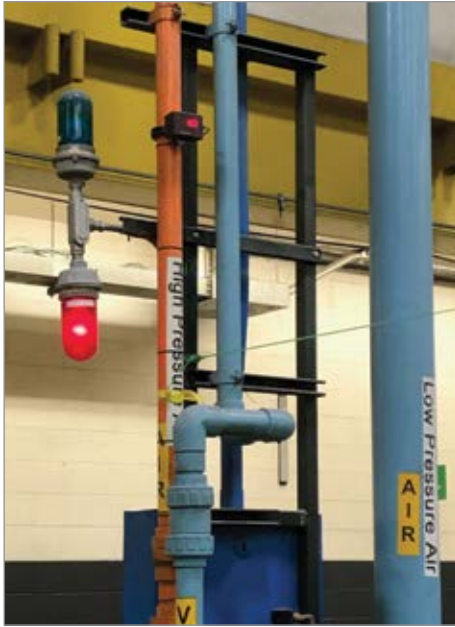
The Sussex plant uses airflow meters on all major pieces of equipment and processes to measure compressed air performance. Shown is an airflow meter on a high-pressure line.
