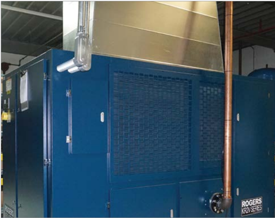
Figure 5: Installed 2-stage enclosed compressor with vertical ductwork
