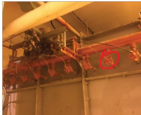
Figure 6. Six reverse pulse dust collectors exist in the facility. The failure of one blast valve caused low pressure in the plant during a final measurement period.
