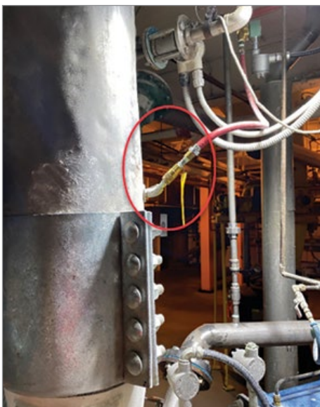
Figure 7. Plant personnel had made modifications to product chutes to prevent clogging, the continuous flow of this blowing represented 15% of the total plant cfm demand.
