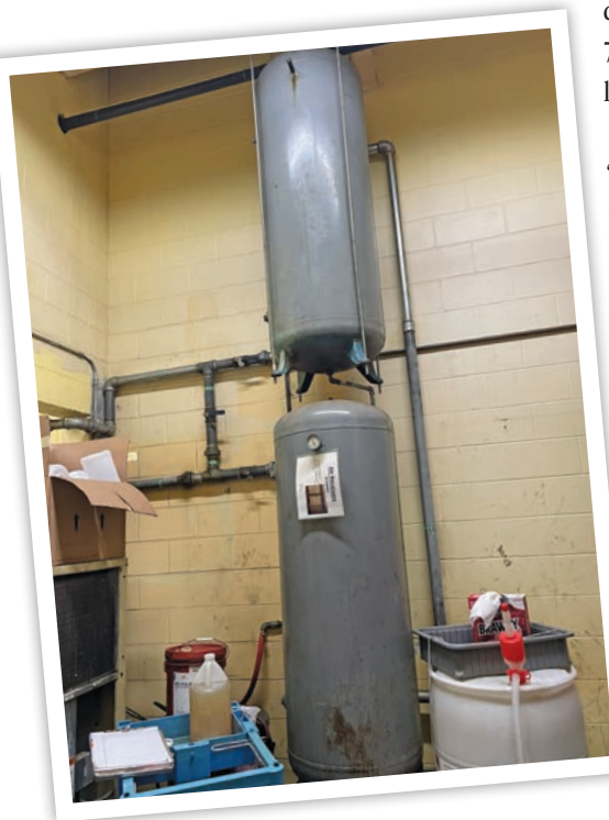
These stacked compressed air storage tanks presented a safety concern.
