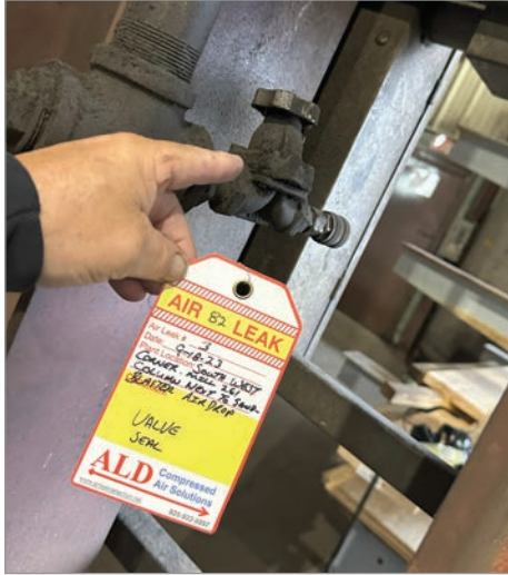
"Before and After" pictures of a compressed air leak at the plant.
