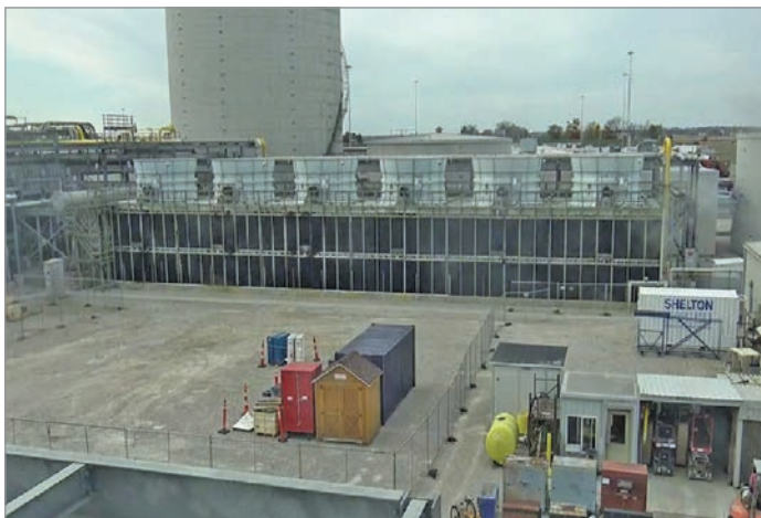
Before: Existing field-erected towers needing to be replaced.
