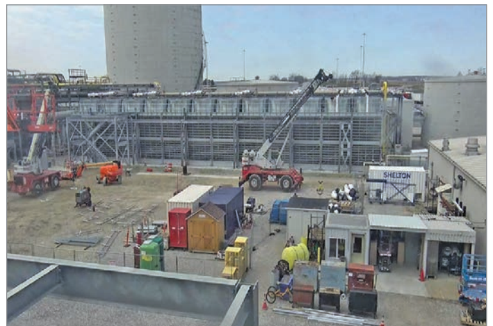
After: The BAC Series 3000 modules were installed in only 4 days, compared to the 2-3 months required to assemble field-erected cooling towers.
