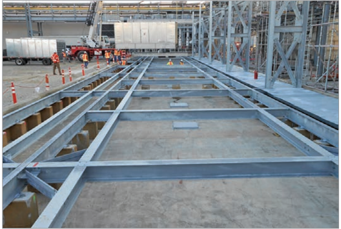
The BAC Series 3000 modules were installed on the existing concrete cold-water basin.
